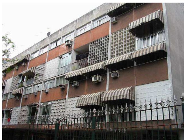
Figura 2. Fachada Bloco B2 (Foto GAP)
