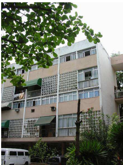
Figura 1. Fachada Bloco B1 (Foto GAP)
