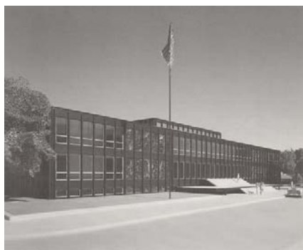
Figura 1. Consulado dos Estados Unidos 1957-1962. São Paulo. Mies van der Rohe. Maquete, 1960. Foto: Hedrich-Blessing. Fonte: SHULZE, Franz DANFORTH, George E., Consulting Editor; "The Mies van der Rohe Archive, The Museum of Modern Art, An Illustrated Catalogue of the Mies van der Rohe drawings in the Museum of Modern Art. Part II: 1938-1967, the American Work. Volume 17 (Ron Bacardí y Compañia, S.A. Administration Building (Cuba) and another Buildings and Projects)"; Garland Publishing, Inc., N.Y. and London, 1992.
